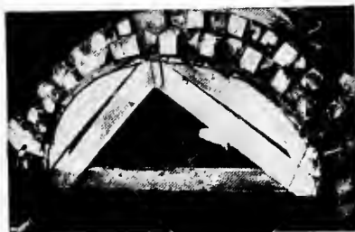
FIG. 127. —Centering for Brick Sewer.
