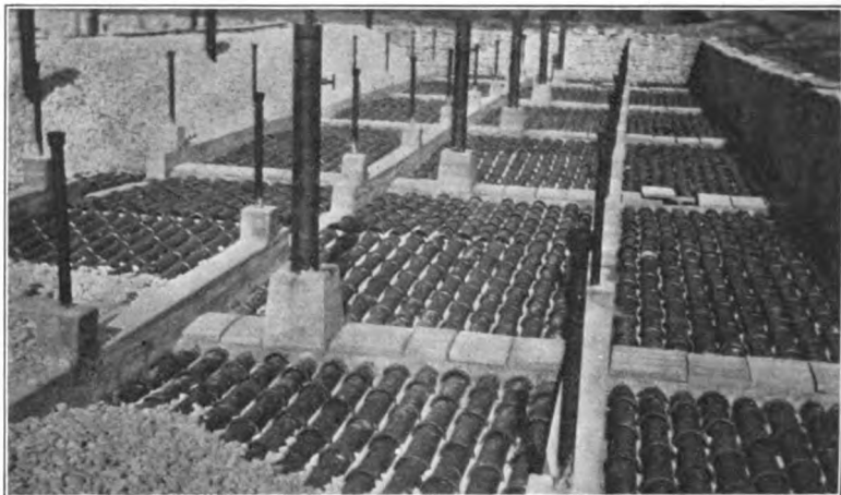
FIG. 69.—Filter floor, Atlanta, Ga.
