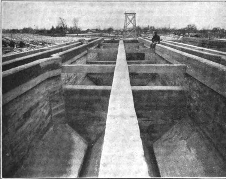
FIG. 40.—Two-story tank at Batavia, N. Y.
