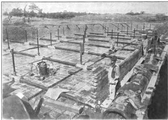
FIG. 70.—Tile filter floor, Batavia, N. Y.
