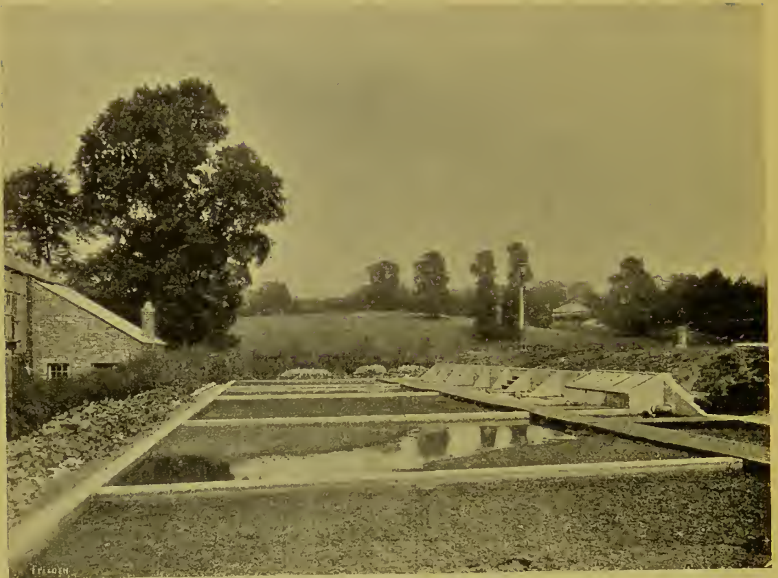
Fig. 31.—EXPERIMENTAL SEPTIC TANK AND FILTERS, BELLE ISLE, EXETER. Diagram of Overflow Pipes.
