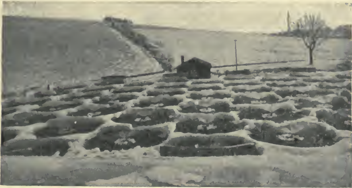
FIG. 47.—View of Sprinkling Filter at Danville, Pa., in Winter.
