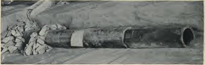
FIG. 31.—Photograph of Tile laid as if for Sewage Disposal.
