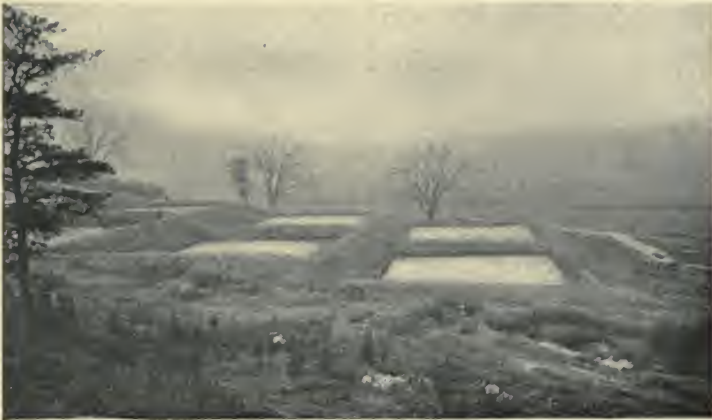
FIG. 37.—View of Sand-filter Beds for Village in Massachusetts.
