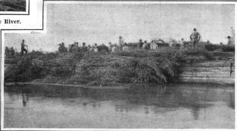
Making Brush Mats for Closure Works.
