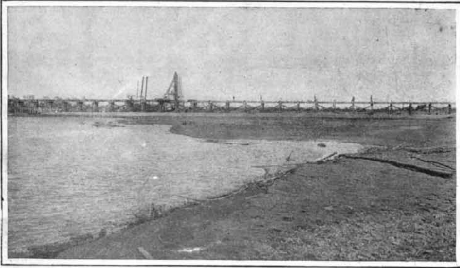
Trestle Over Hind Dam, Lower Heading.
