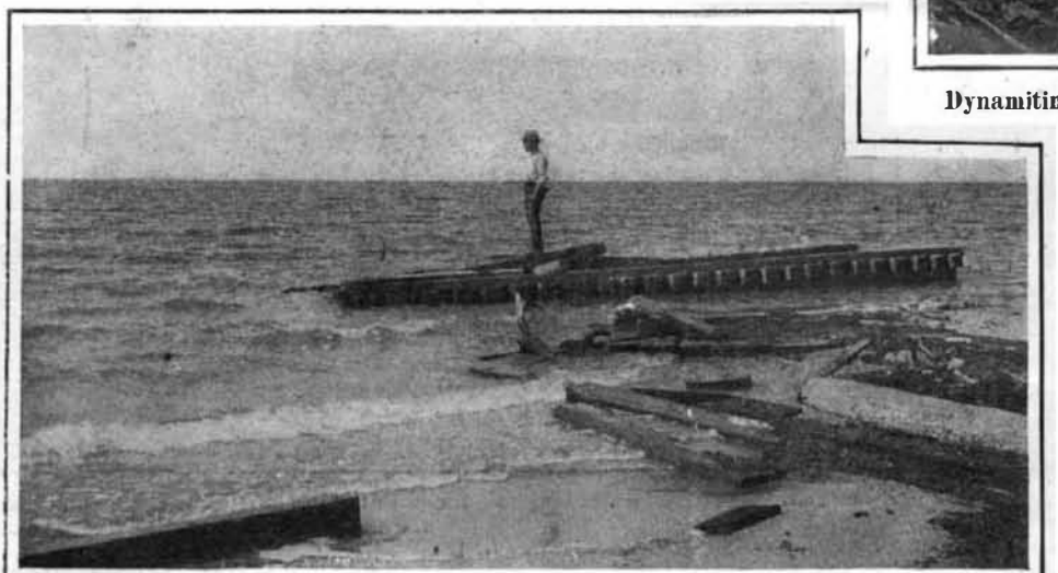
Railroad Wreckage on the Shores of the Salton Sea.
