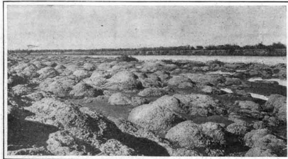
New Bed and Channel of the Colorado.
