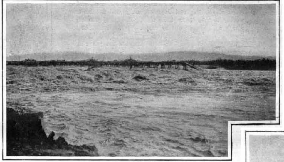
The Washing Away of a Trestle.
