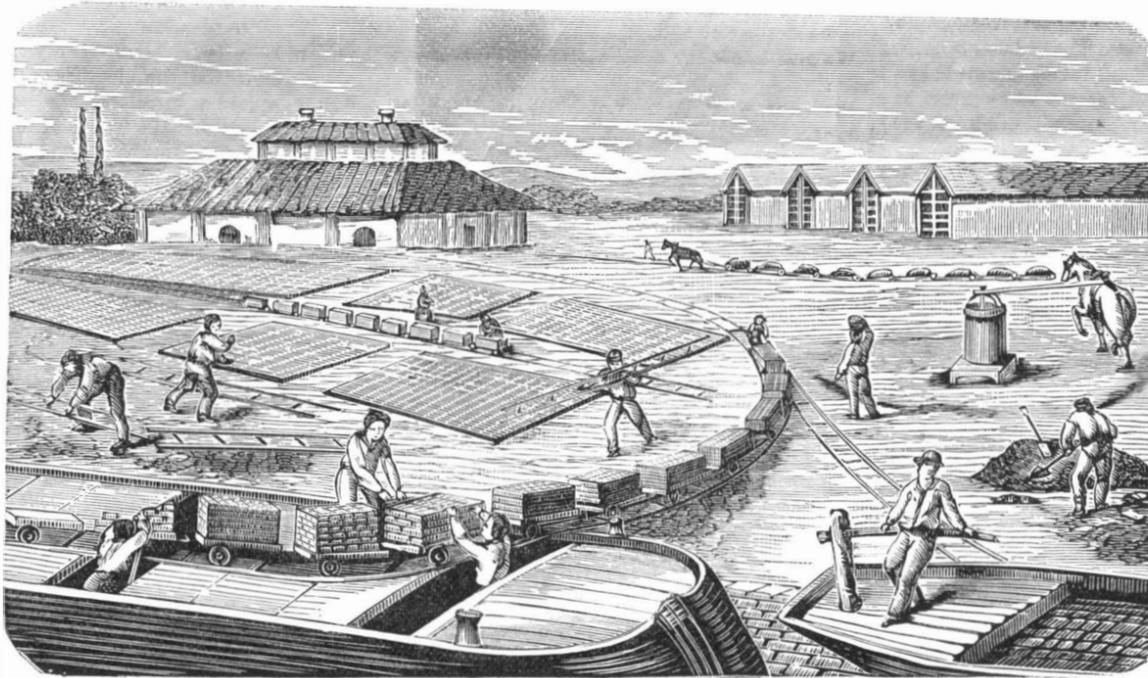
**PORTABLE RAILWAY IN A BRICKYARD.**
