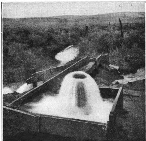
FIG. 8. — A FLOWING OR TRUE ARTESIAN WELL.
