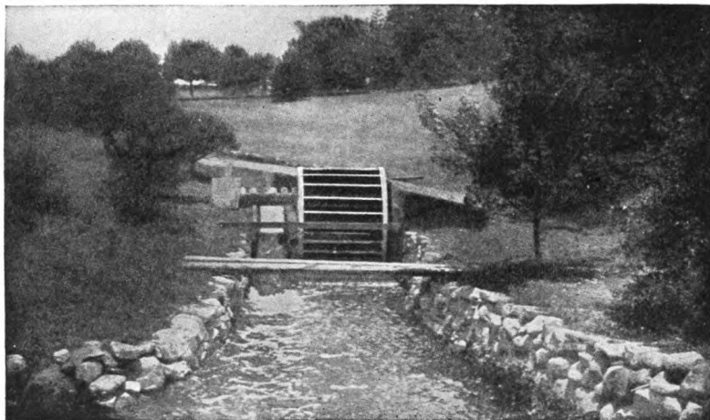
FIG. 16. — DOWNSTREAM VIEW OF WATERWHEEL USED FOR PUMPING WATER.
