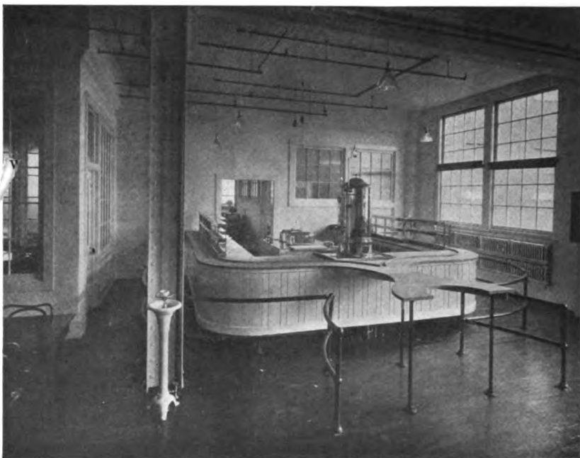
Courtesy National Lamp Works.
