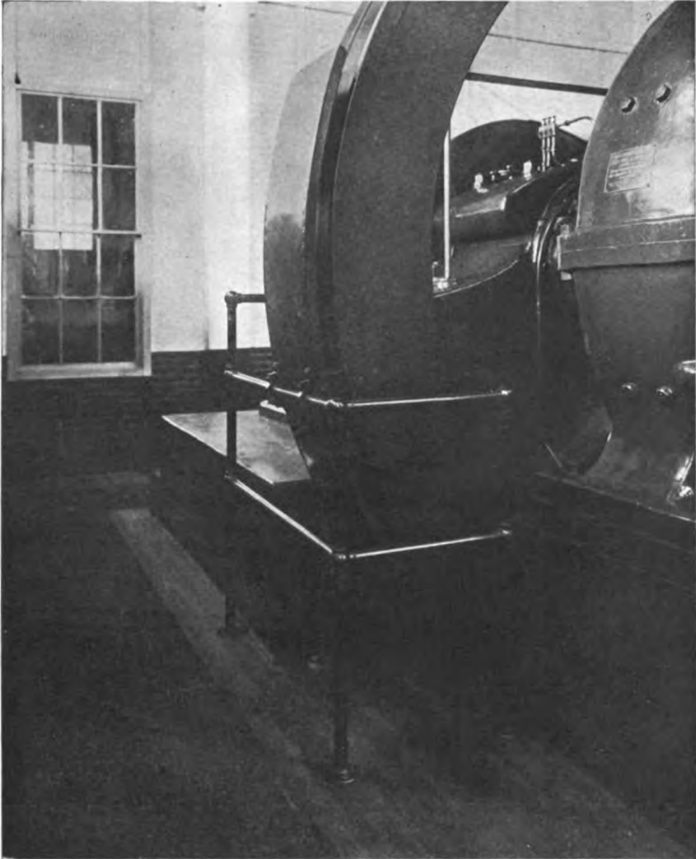
Guard in Front of Fly Wheel.
