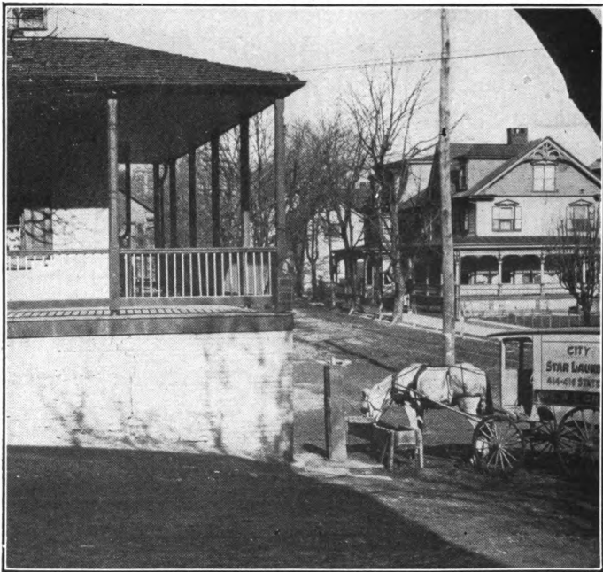
FIG. 38.—The Town Pump—a thing to be avoided. (Photograph by the Author.)
