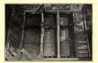
FIG. 18.—BIRD'S-EYE VIEW OF EXPERIMENTAL SEPTIC TANKS F, G, AND H DOSED WITH CITY SEWAGE
