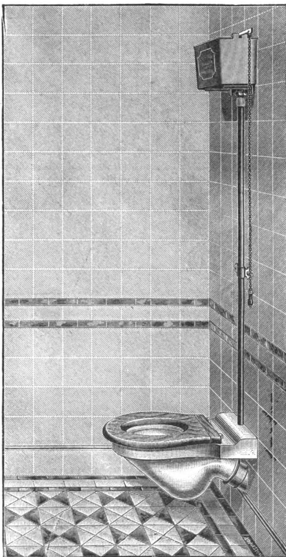
FIG. 193.—Corbel water-closet complete.
