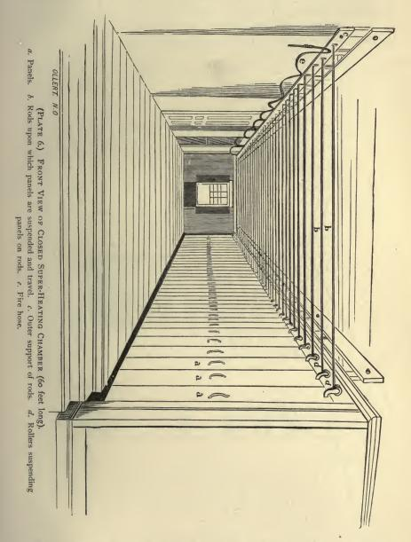
nails, or better, by nails supplied with tin discs or washers, a double layer of "Asbestos Building Felt," well lapped and securely tacked, thus rendering the interior of the chamber fire-proof.
