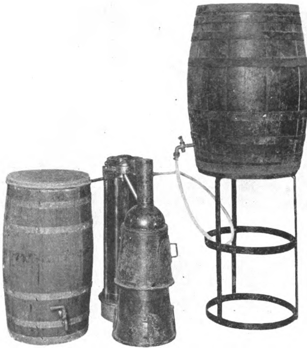
Fig. 19.—Forbes' sterilizer with "wood-burning attachment" and "barrel accessory."
