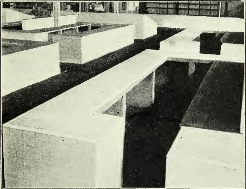
FIGURE 23.—Rat-proof market stalls. Rats are unable to climb the smooth tiles to get at foodstuffs left on the counter
