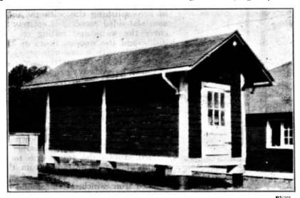
FIGURE 9.—An inexpensive method of rat proofing a corncrib. It is supported by glazed tiles capped with galvanized washtubs, which, though not attractive in appearance, have successfully kept out rats
