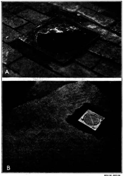
FIGURE 17.—A, Broken floor drains provide a ready means for invasion by rats; B, rat tracks in fresbiy laid concrete around newly repaired drain show that before repairs were made the drain was a rat highway
