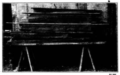
FIGURE 2.—Lumber and other stored materials piled weil off the ground to prevent rat harborage
