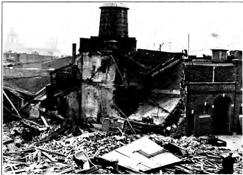
FIGURE 1—A building wrecked when the welded head seam of an ammonia generator failed injuring a man and causing $15,000 property damage. An illustration of the kind of accident that for years postponed acceptance of welding as reliable for pressure vessel construction.
