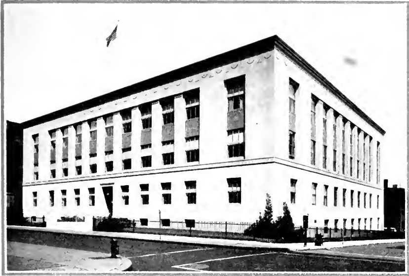
GENERAL VIEW— Showing the results obtained by the architect in using a modern classic design to produce a building of striking simplicity and beauty. In relief on each of the spandrels between the upper rows of windows are intertwined a gear and a governor, suggestive of the Company's business.
