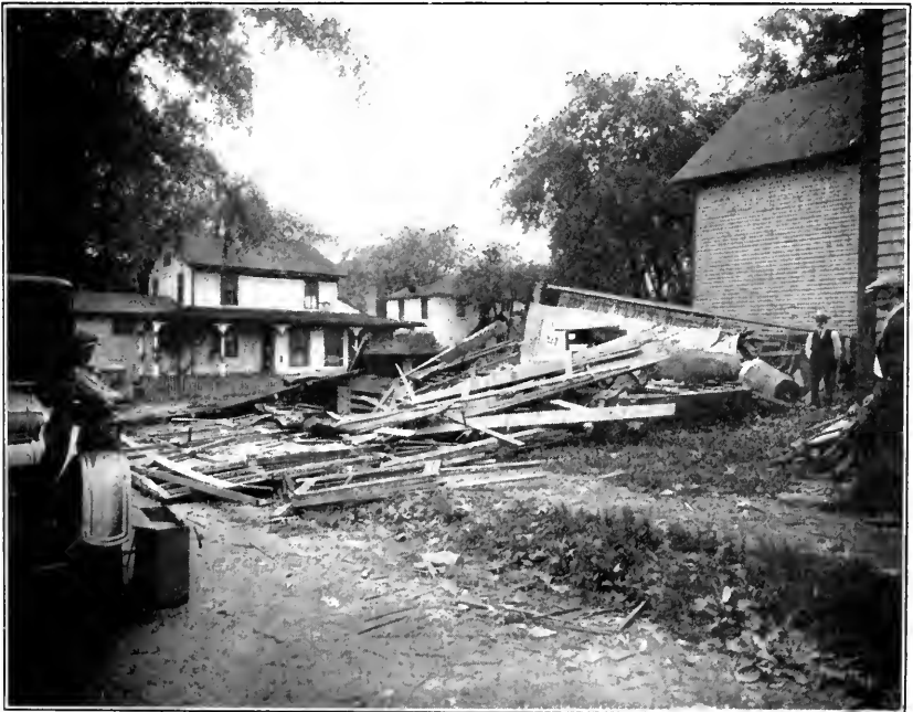
HOT WATER SUPPLY TANK EXPLOSION AT WATERVILLE, CONN.
