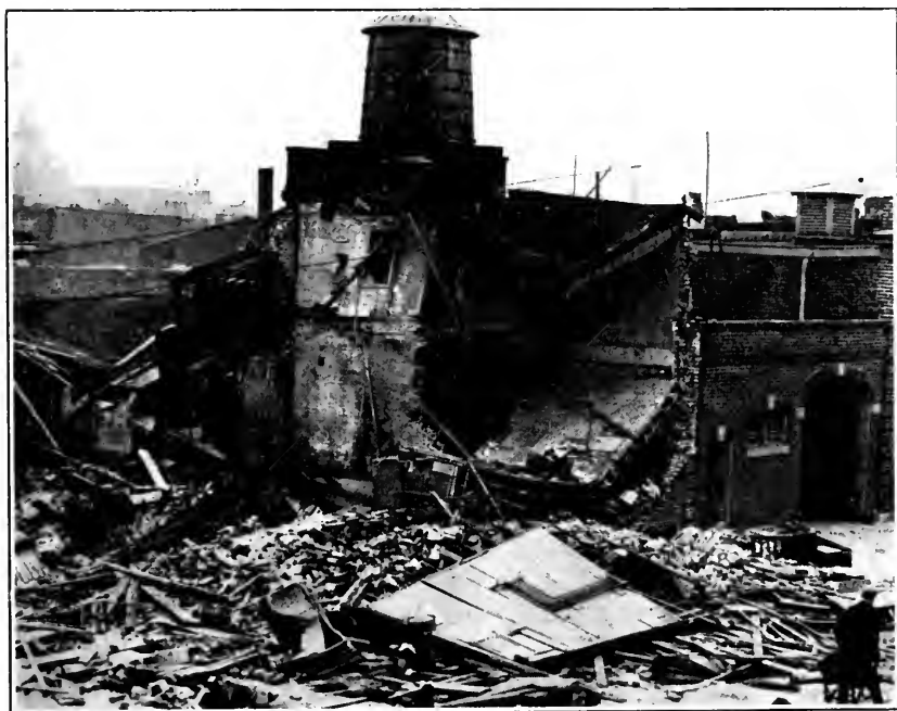
AMMONIA GENERATOR EXPLOSION AT PHILADELPHIA, PA.
