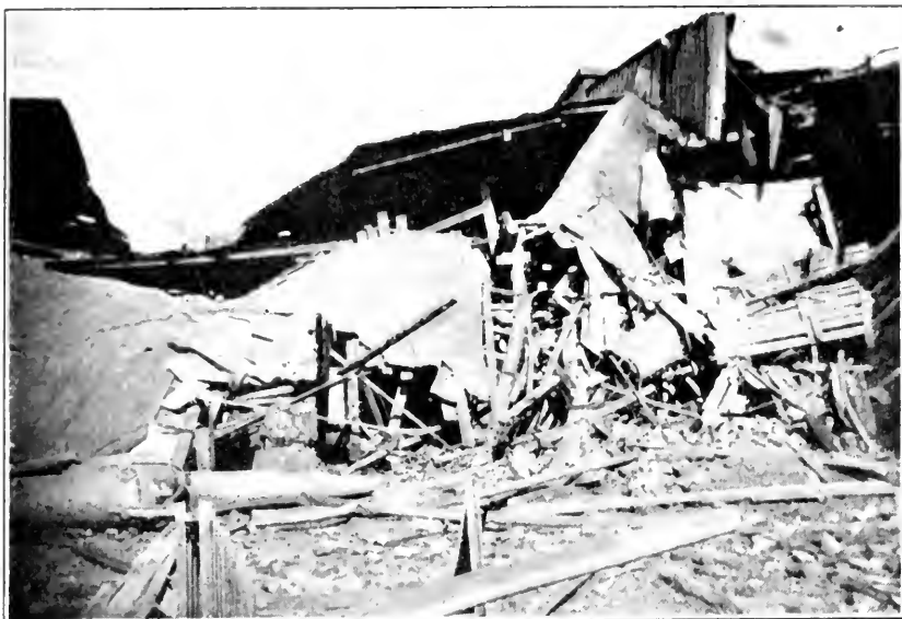
Excessive internal corrosion in a horizontal tubular boiler at a brick yard in Richmond, Va., caused the explosion shown above. The accident demolished the building and wrecked an engine, causing property damage of almost $10,000.
