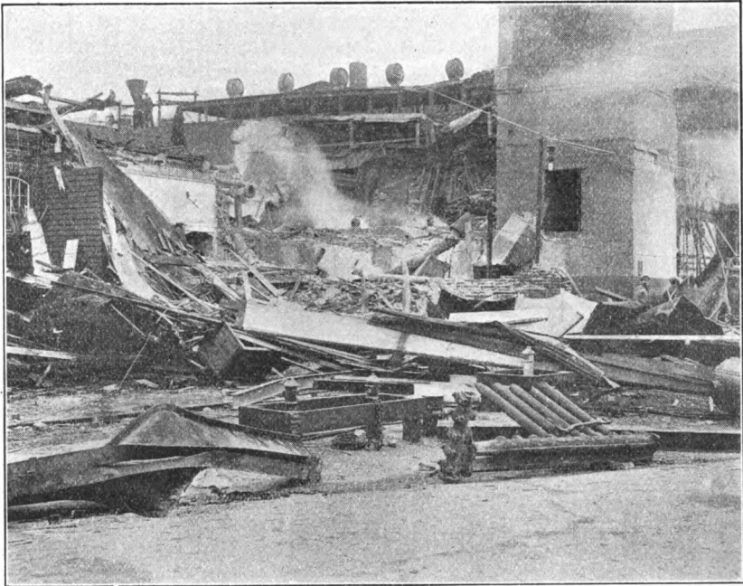
FIG. 4. SHOWING PORTIONS OF THE NO. 2 ECONOMIZER STANDING ON ITS PLATFORM JUST BACK OF THE STACK.
