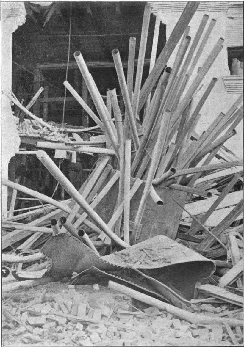
FIG. 2. COURSE "E" AND ITS LOAD OF TUBES.
