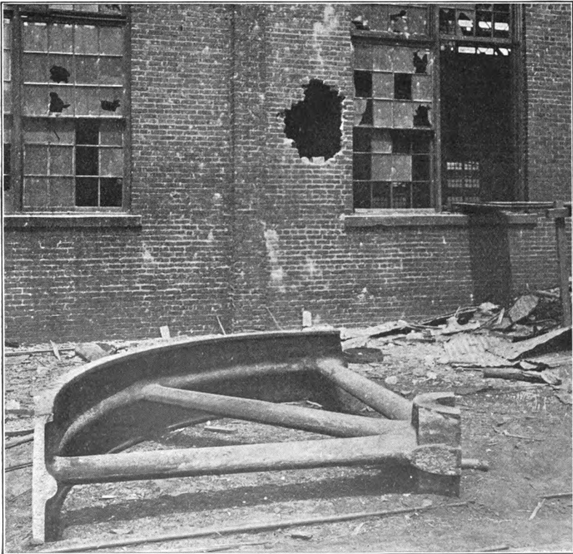
AN UNUSUAL FLY-WHEEL BREAK. BIRMINGHAM, ALABAMA.
