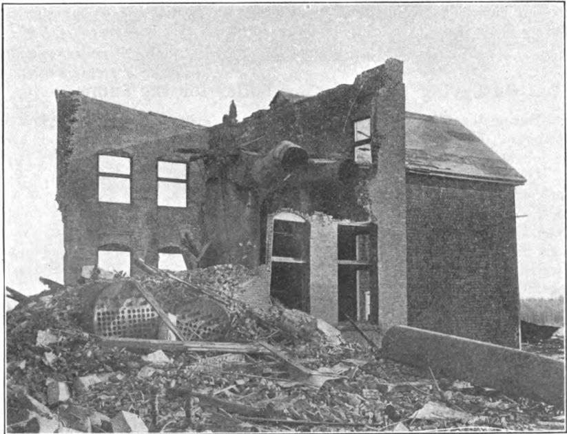
FIG. 4. WRECKED BOILER HOUSE.
