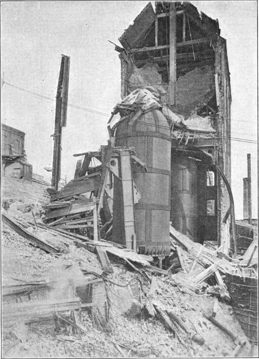
FIG. 2. VIEW LOOKING INTO THE WRECKED DIGESTER HOUSE.
