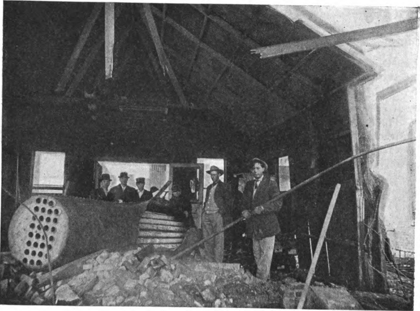
THE BOILER WHICH DID NOT NEED INSURANCE.
