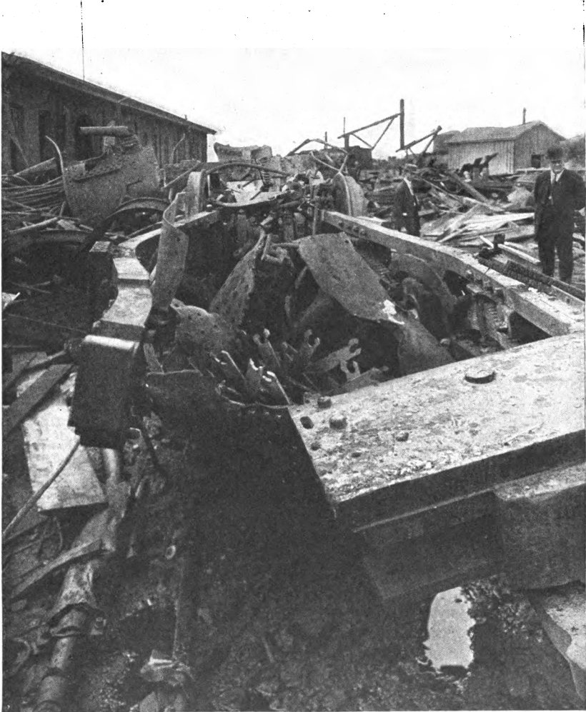
FIG. I. SHOWING BROKEN SLING STAYS.
