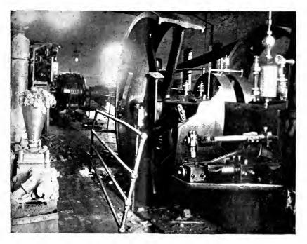
FIG. 1.— SHOWING THE BROKEN WHEEL AND GOVERNOR.
