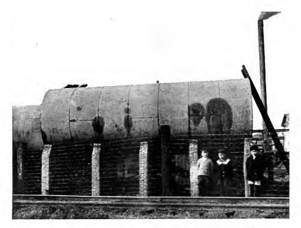
FIG. 2. THE PATCHED OIL TANK.
