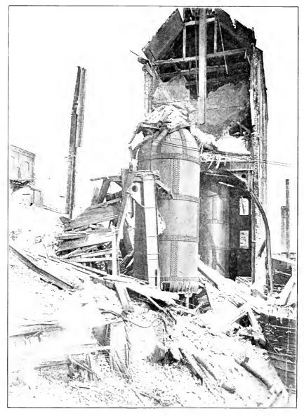
FIG. 2. VIEW LOOKING INTO THE WRECKED DIGESTER HOUSE.
