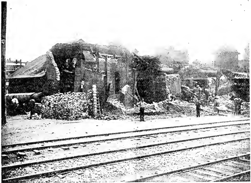
FIG. 3.—GENERAL VIEW OF THE DESTROYED POWER PLANT.
