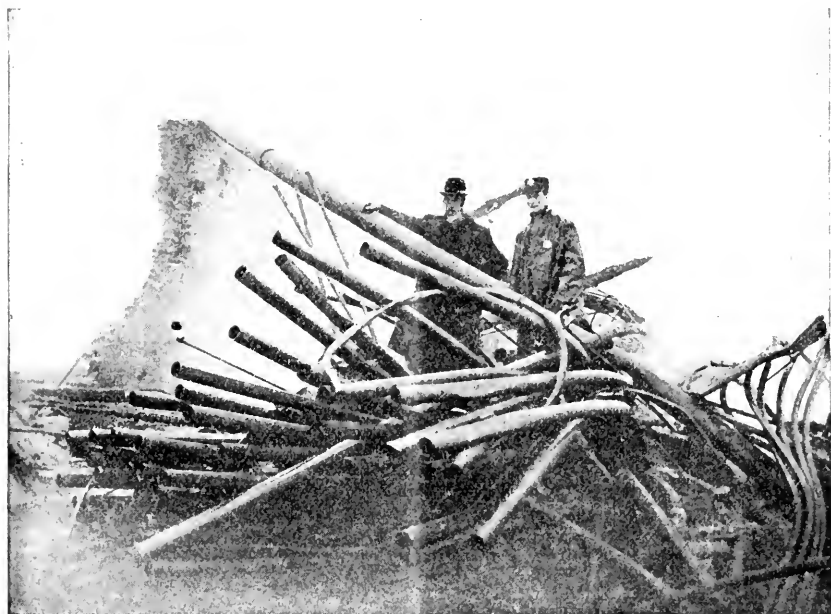
FIG. 5. — SHOWING THE TUBES OF THE EXPLODED BOILER.
