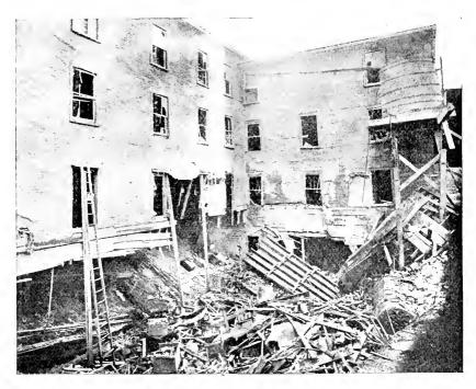
RUIN WROUGHT BY THE EXPLOSION OF A HORIZONTAL TUBULAR BOILER.
