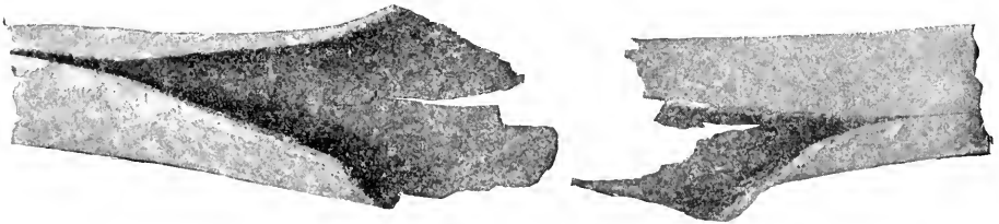
FIG. 2. — ANOTHER VIEW OF THE SAME PIPE.
