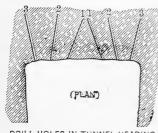
DRILL HOLES IN TUNNEL HEADING
