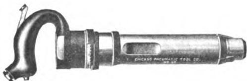
Fig. 4979. "Boyer" Riveting Hammer.
