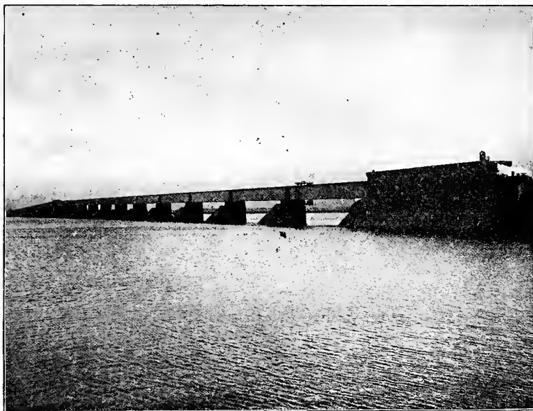
Old Victoria Tubular Bridge Over the St. Lawrence, Grand Trunk Railway, Montreal, Canada
