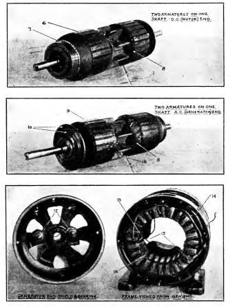
FIG. 122 (continued).-Motor-generator set of Fig. 121 partly dismantled.
