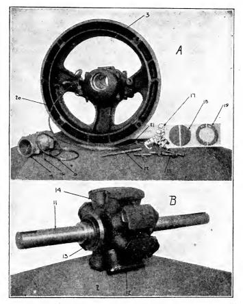
FIG. 101-A-B (C and D on opposite page).—Alternating-current generator, 150 KVA., 900-R. P. M., 60-cycle. Single phase. Dismantled parts listed below.
