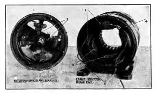
FIG. 122 .- Motor-generator set of Fig. 121 partly dismantled.
