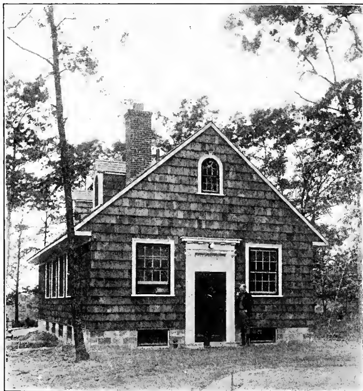
FIG. 179.—The house in which the Radio Corporation has all its receiving sets for trans-Atlantic communication. All the commercial trans-Atlantic stations in Europe are received by instruments in this house, using one antenna.
