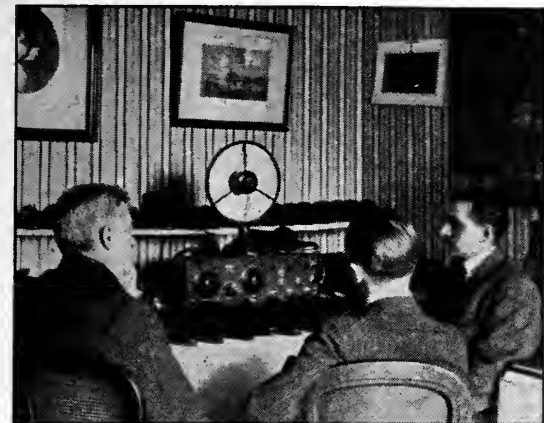
A progressive New York shoe salesman has installed a radio receiving set to entertain his customers. The large conical device is a loudspeaker made with a parchment diaphragm which reproduces music with little or no distortion
