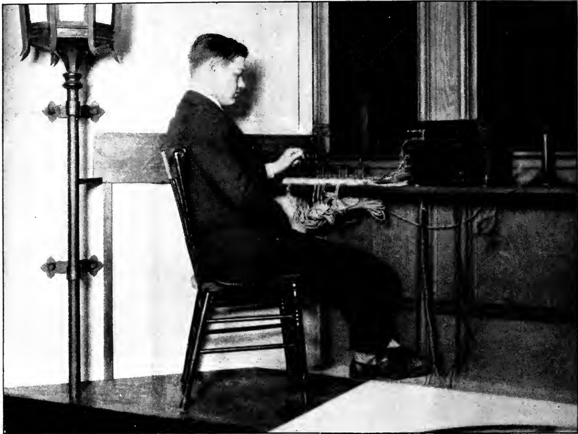
Amplifying box and switches leading to the various microphones located in different parts of Calvary Church. An operator (in this photograph, W. W. Rodgers, author of this article) sits up with the choir, and throws the switches to open the proper microphones at the right times
