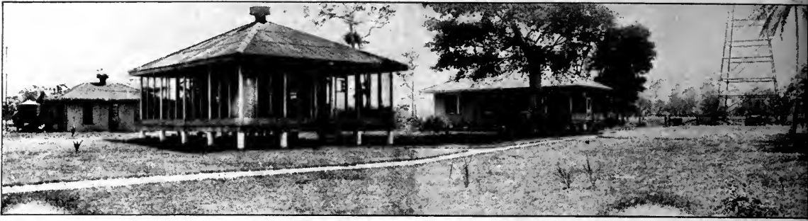
THE RADIO STATION AT TELA, HONDURAS
