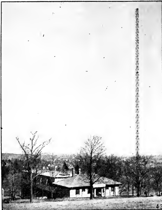
THE FIRST TOWER AT WGI
