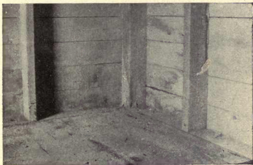
The flooring must be perfectly tight to prevent drafts coming through it
