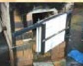
The last thing I do is to make up a mixture of equal parts of scrap clay, sand, and sawdust. Initially this is used to fill up any cracks or unevenness in the joints between the bricks. It can also be used as an insulating layer on the outside of the kiln. You can see some evidence of its use in the last picture on the right. I also use it as a seal between the pot chamber and the thick shelves that make up its lid.
