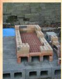
Here you can see the 3 channels which are the primary air entries in this design. The channels extend right through to the other end to provide enough for full combustion (see the notes on proportions at the end of this section). During firing one or more entries can be closed at either end to help vary the atmosphere inside.
