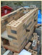
This has now reached the stage where the firebox is complete and the pot chamber and base of the chimney can be built. Notice that the last layer of bricks has been corbelled in to support the base shelves. Notice also the gap at the end of the shelves to allow fire entry from the firebox. In this case it is about
