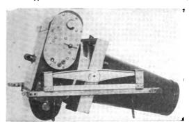
Fig. 93.-U. S. type "K" film camera on universal mounting, oblique position.
