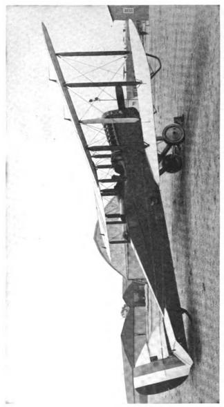
Fro. 100.—DeHaviland 4 re-constructed as a special photographic plane, showing 20-inch camera mounted for oblique photography.
