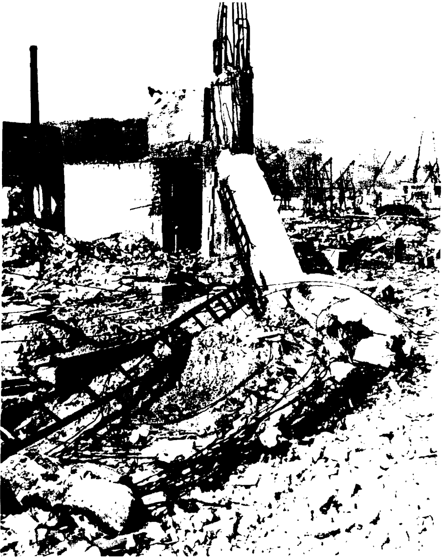
Figure 5.34b. A circular, 60 feet high, reinforced-concrete stack (0.34 mile from ground zero at Hiroshima). The failure caused by the blast wave occurred 15 feet above the base.
