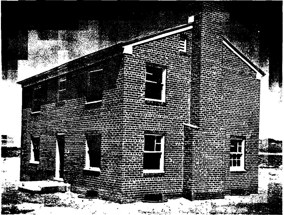
Figure 5.68. Unreinforced brick house after a nuclear explosion (1.7 psi peak overpressure).
