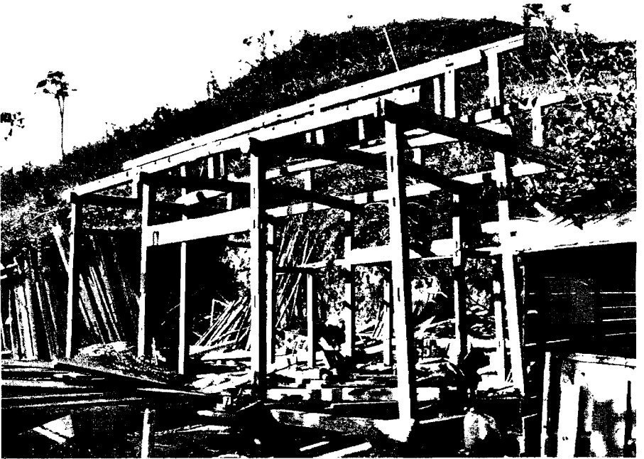
Figure 5.52. Upper photo; Wood-frame building; 1.0 mile from ground zero at Hiroshima. Lower photo: Frame of residence under construction, showing small tenons.
