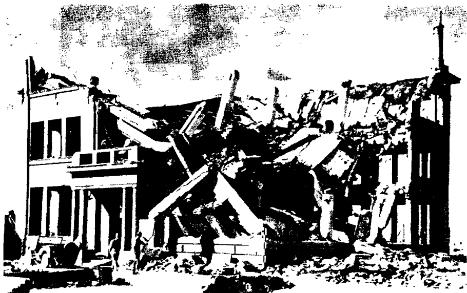
Figure 5.20b. Three-story, reinforced-concrete frame building; walls were 13-inch thick brick panel with large window openings (0.13 mile from ground zero at Hiroshima).
