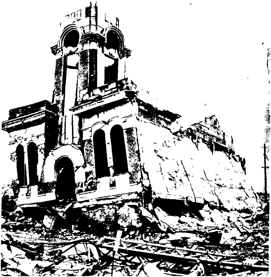
Figure 5.26. Two-story, steel-frame building with 7-inch reinforced-concrete wall panels (0.40 mile from ground zero at Hiroshima). The first story columns buckled away from ground zero dropping the second story to the ground.
