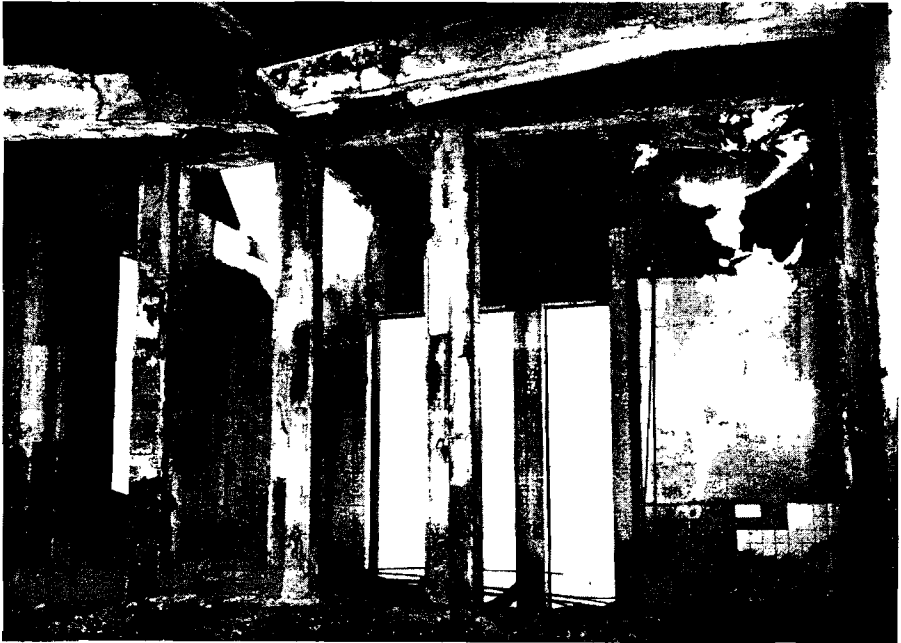
Figure 5.20a. Upper photo: Reinforced-concrete, aseismic structure; window fire shutters were blown in by blast and the interior gutted by fire (0.12 mile from ground zero at Hiroshima). Lower photo: Burned out interior of similar structure.
