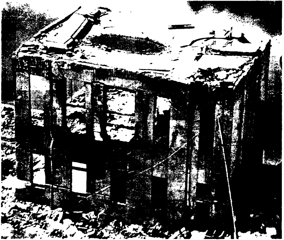
Figure 5.22a. Depressed roof of reinforced-concrete building (0.10 mile from ground zero at Hiroshima).
