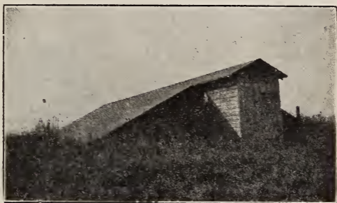
Old Shed in Paterson, N. J., used for a Mushroom House by Mrs. Thomas Smith, supporting herself and five children.
