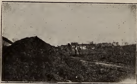
Pile of Material ready to be drawn to Mushroom Houses.
