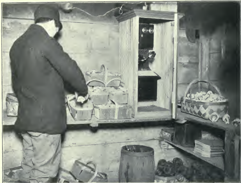
FIGURE 238.—View in packing room, Akron "tunnel," N. Y. Mushroom Co.; placing mushrooms in basket. Copyright.
