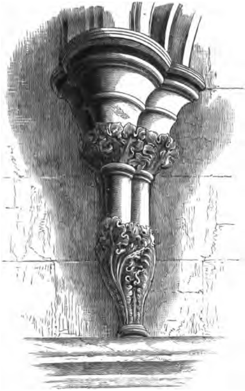
Corbel in the North Aisle.
