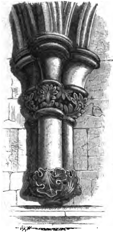
Corbel in North Aisle.
