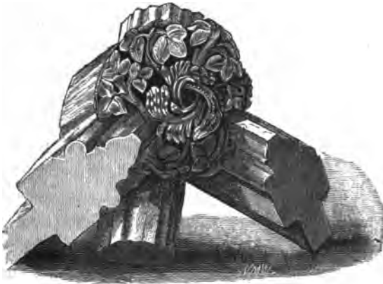
Curious Key-stones of Moulded Ribs of Groined Arches, from the Wax Cellar.
