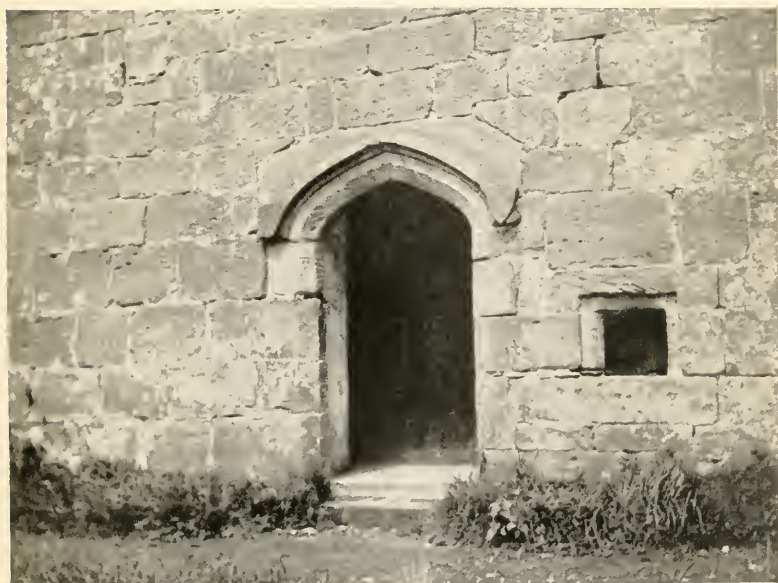
CELL DOOR AND HATCH, GREAT CLOISTER. MOUNT GRACE.
