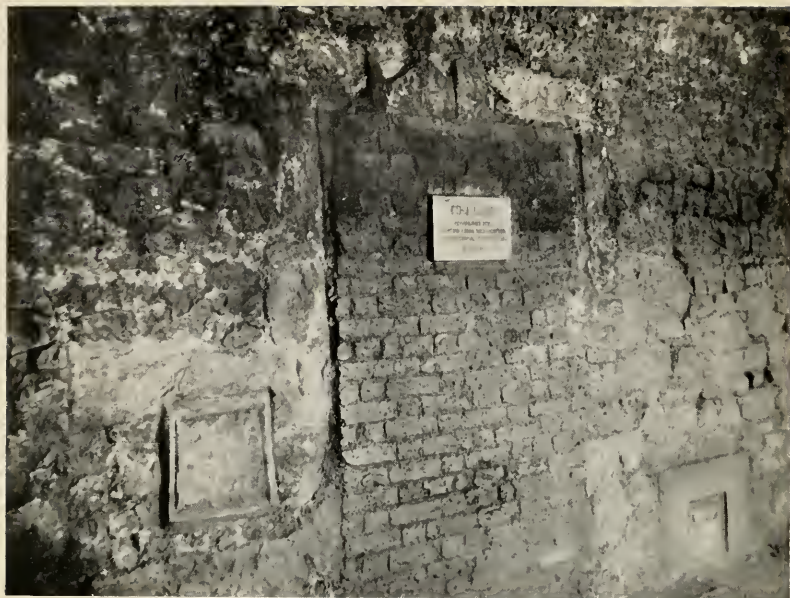
DOOR OF B CELL: WEST WALL OF GREAT CLOISTER. 1371.
