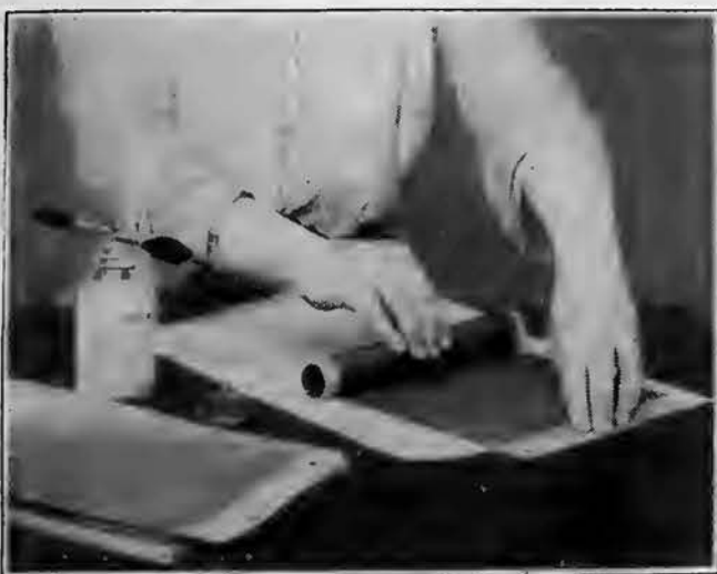
Method of smoothly relaying the Stencil Sheet
