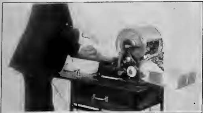
Hand feeding the electrically driven Mimeograph
