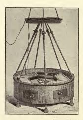
FIG. 215.—Batut's kite for photographic apparatus.
