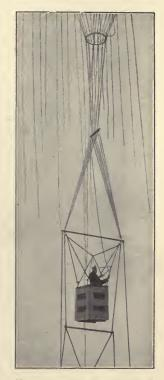
FIG. 94.—French method of suspending the basket for an observer.
