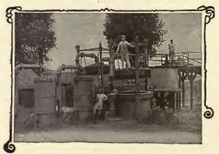
FIG. 92.—Old method of generating hydrogen.
