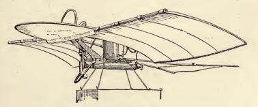
FIG. 58.—Hofmann's first model with carbonic acid motor.
