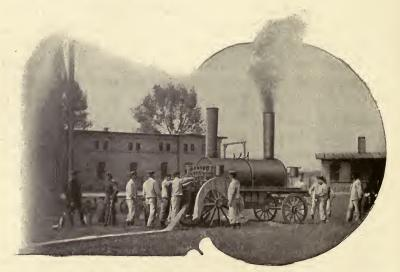
FIG. 88.—Steam winch for pulling in a captive balloon. (From "Die Geschichte der Luftschiffer-Abteilung.")
