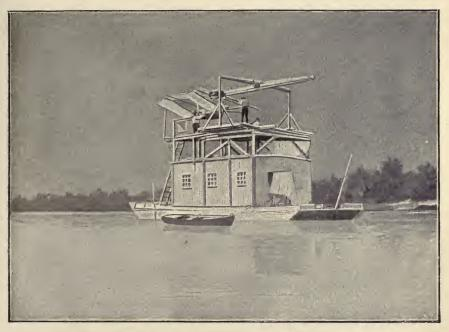
FIG. 56.—Starting arrangements for Professor Langley's flying machine.
