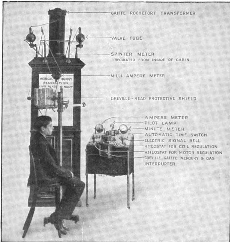
FIG. 338.—A convenient arrangement of apparatus for therapeutic work.
