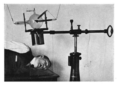
FIG. 22.—Position for lateral röntgenography of head.
