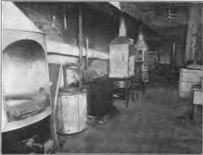
Fig. 2. Hardening Plant, Wheelock, Lovejoy & Co., looking toward Street
