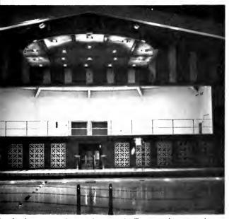
ershey's new outdoor-indoor pool. Two southern quadrants wall roof section are morable. Two 2-horsepower, two-speed ear motors drive each section. It takes approximately
