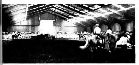
Some of the world's finest quarter horses train in this pre-engineered building at Westernhook Farm, Southbury, Connecticut. The rigid frame-type construction permits a trainin area without obstructions.
