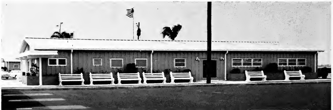
Clearwater Lawn Bowling Club, Clearwater, Florida. Armco Building in background provides lounge and meeting facilities for members. Dealer: Mathews Development Corporation, Tampa, Florida.
