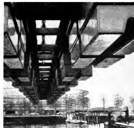
Looking underneath Fiberglas-reinforced plastic prefabricated pontoons set in a wood framework to form prototype header.
