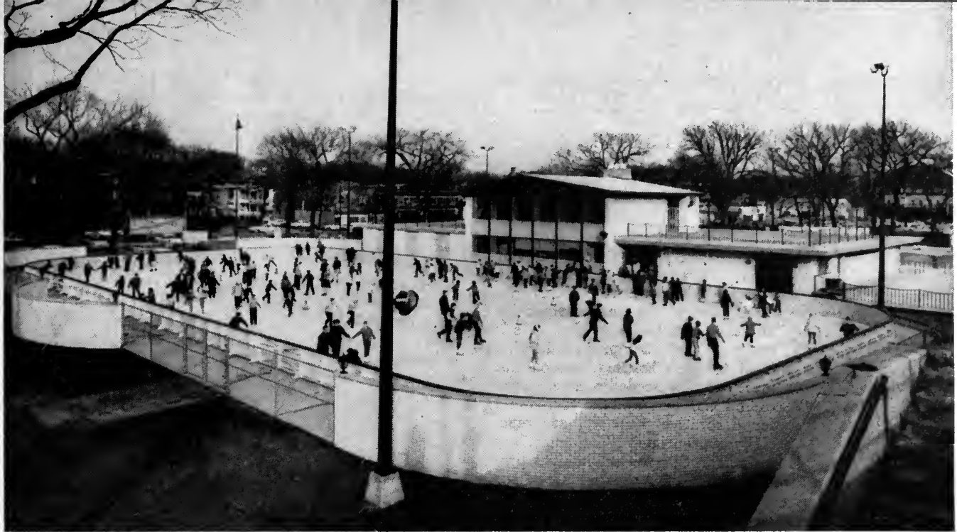
Ideally, thirty square feet of ice should be allowed for each person skating.
