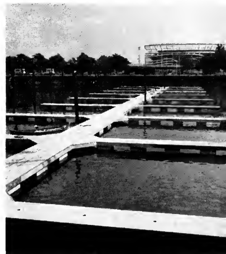
Advantages of this Fiberglas flotation system: headers and fingers are kept at a constant level in relation to the boats.
