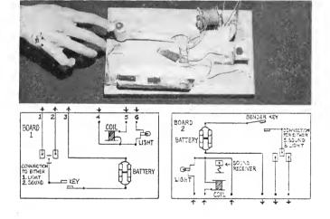
This set could be made and used by any hospital patient who has free use of his hands. The key is constructed so that a message can be sent by either sight or sound. Two boards should be made in order for two persons to receive and send messages back and forth. To transmit to another key, wires would be connected to the batteries and the light. To send by sound, a wire would be connected to the coil.
