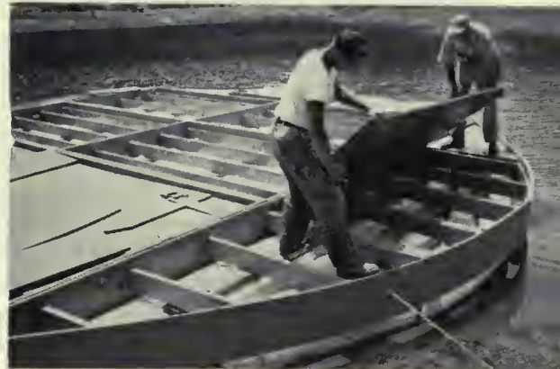
Wooden framing is then covered with plywood. Note side rope holds anchor.
