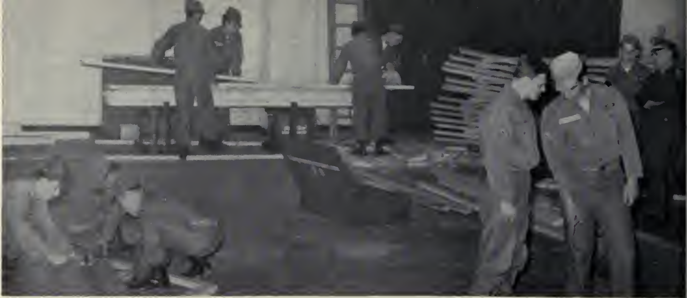
Shelters were partially assembled in the reserve training center. Reservists on the floor in the left foreground are assembling part of the shelter. In the background men are sawing wood for the shelters. On the right, two privates are discussing next step in the operation; behind them a staff sergeant and captain drop in to survey the project, see how it's going.
