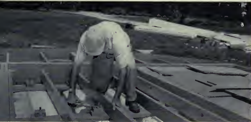
In the third phase of building, wooden sections and planks are joined to the Dow Styrofoam log flotation material.
