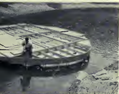
Nearly finished, island has free-form shape. Final cost of building the 40'-by-30' area: $1500.
