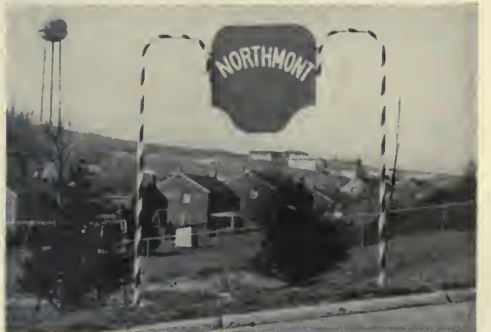
Here is a completed shelter at Northmont. Reservists were all members of Company A 326th Construction Battalion, stationed at Greensburg. The project began in 1958, was finished in time for use in summer of 1959.
