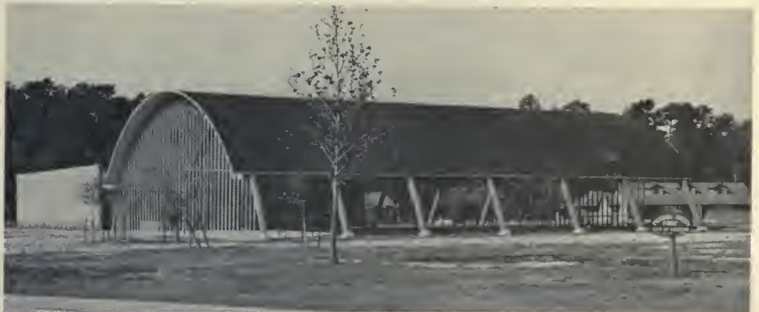
Another 1959 center has Quonset roof, slatted ends, is open on sides.
