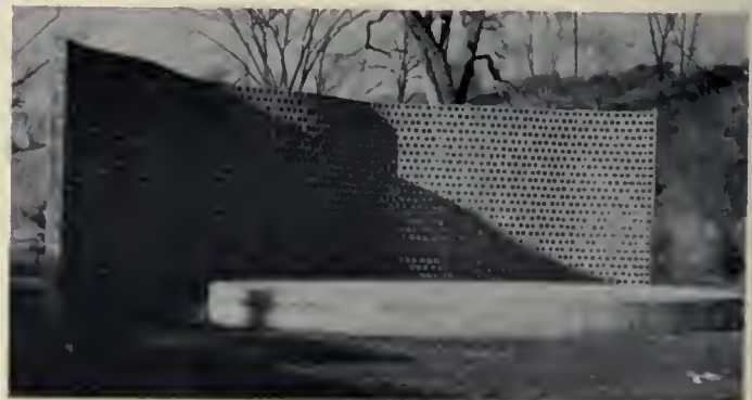
This bandshell, designed for a Lambertville, New Jersey, recreation field by Jules Gregory, is constructed from cinder block, called "partition" block, 6"-by-8"-by-18". The red anthracite cinder gives it an oyster color. The concrete platform is elliptical in shape, forming a concentric relationship to the wall used by the town and its schools for concerts, pageants, and graduations. The ten-acre field of this historic town has ballfields, tennis courts, and park area equipped with picnic tables and fireplaces.
