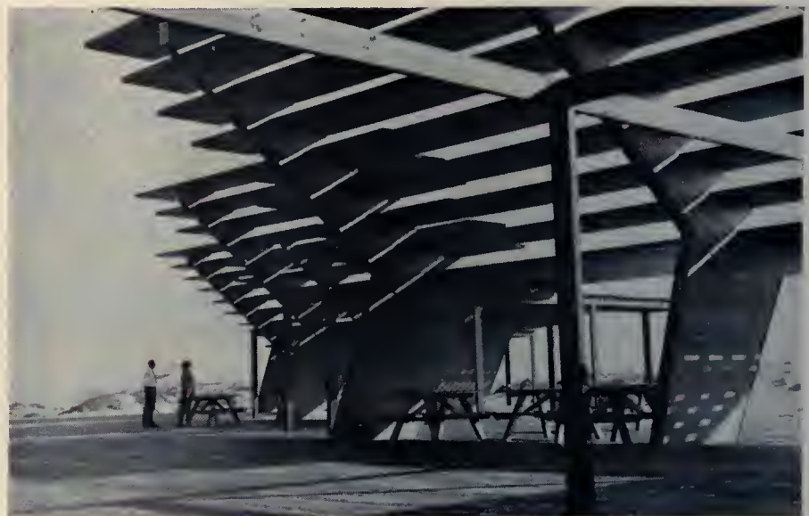
Above are the striking bathing and picnicking facilities at Nags Head, North Carolina. The most dramatic design element is the use of cantilevered fins allowing wind passage but preventing sun passage. Structure was designed for the Cape Hatteras National Seashore Recreation Area by the National Park Service Division of Design and Construction.
