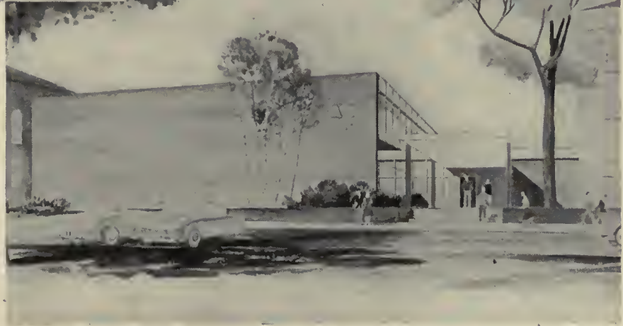
New $751,000 pool now replacing it will double the swimming program.
