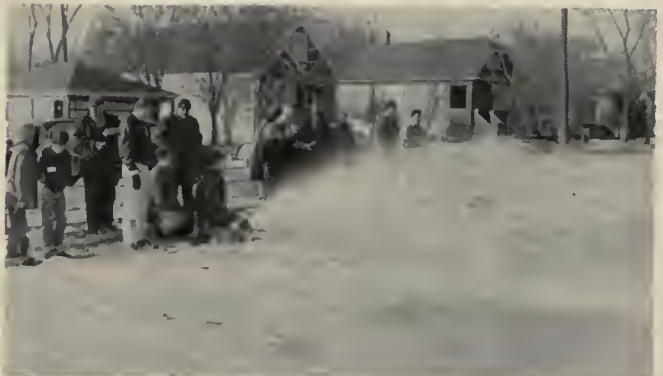
Above: Water must be flooded in immediately as a gust of wind might pick up and tear the light plastic sheet. After area is partially flooded, it is allowed to freeze. Berm was later covered with additional two inches of limestone saturated with water and frozen hard to protect the plastic from skate blades. Subsequent snows and shoveling add to layer.
