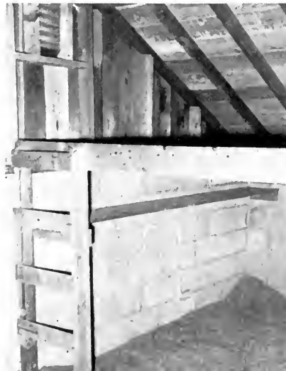
Bunks in each shelter can accommodate ten or twelve campers, are filled with clean sand. Floors are concrete.
