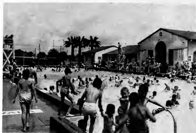
Los Angeles 60 by 120-foot rectangular pool has deep water section across center. Photograph illustrates comparatively heavy use of shallow end sections and the need for wide decks.
