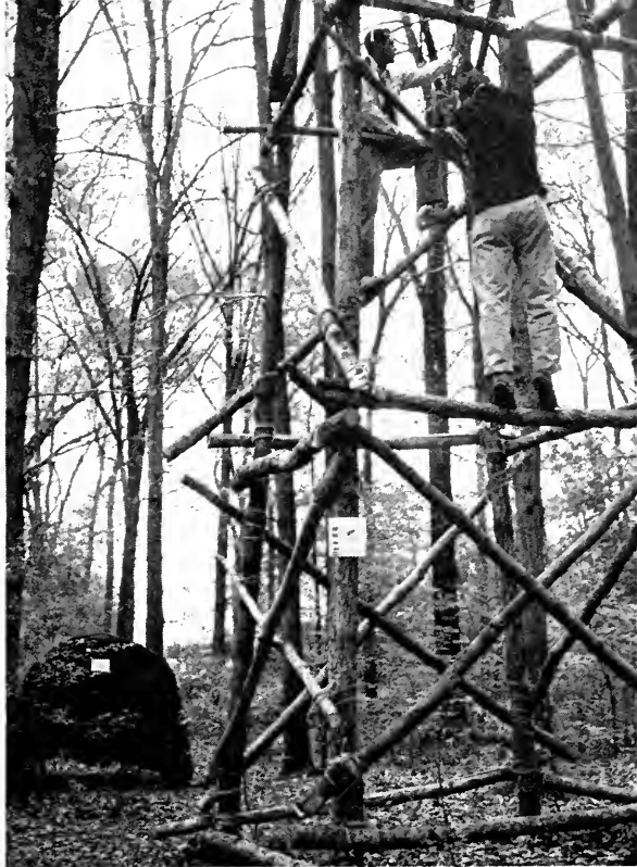
OBSERVATION TOWER. Lashing the structures together made for easier dismantling. Since structures were not permanent in nature, they gave the camp a fair degree of mobility.
