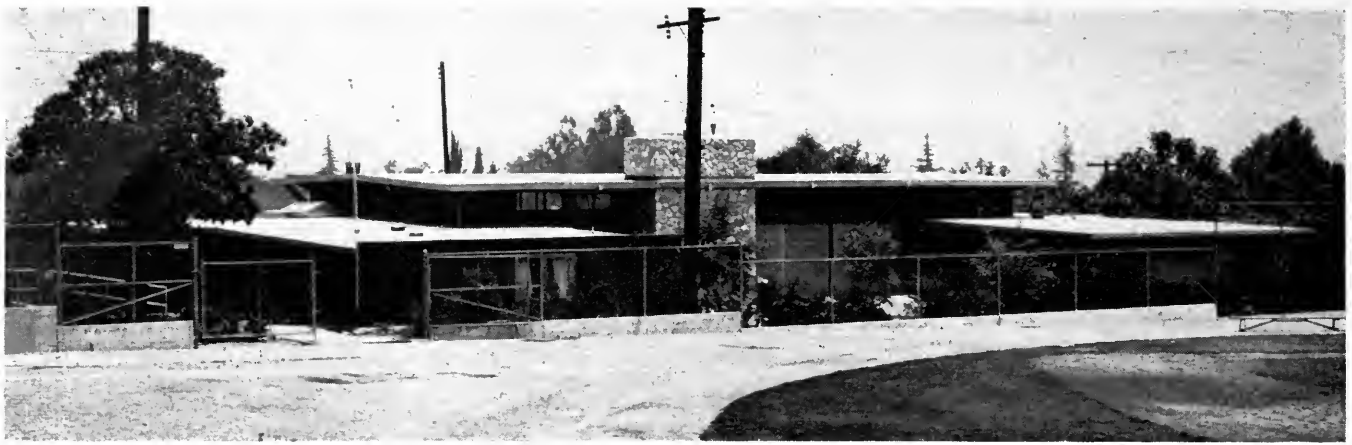
The finished house. Youngsters from junior high school next door enter directly from school grounds in foreground. Sixty-eight car parking lot on left.
