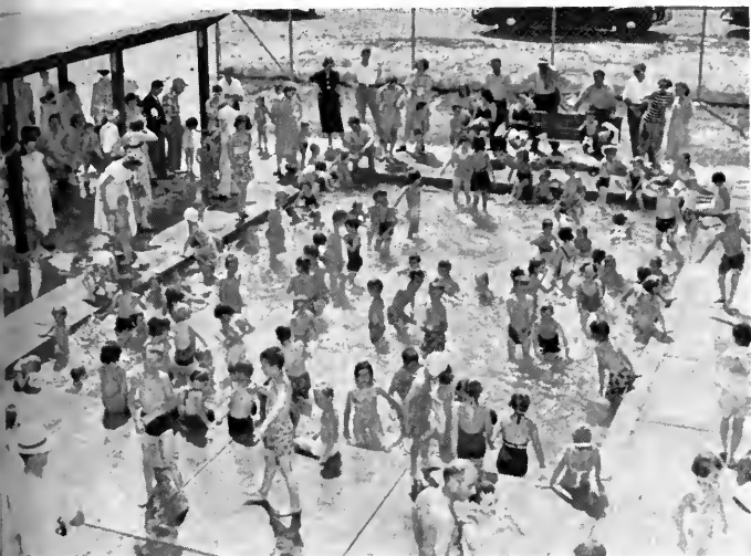
Spring day view of wading pool adjoining Barre, Vermont, swimming pool. Dimensions: 20 by 30 feet; 6 to 18 inches deep. Note shelters and benches for watching mothers.
