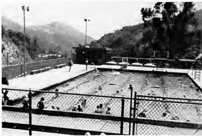
Equipment shown in this view of Hollywoodland Girls Camp Pool, 82½ by 42 feet, includes filters, lights, diving boards and platforms, lifeguard chair and clearly seen line markers.
