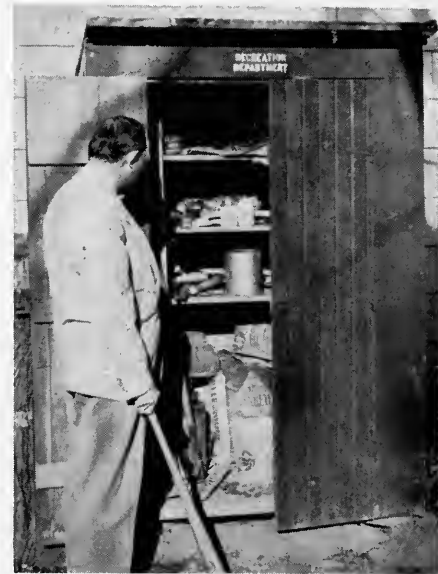
Sheds can be moved by a truck, are set between posts to prevent tipping. Each shelf is designed for certain equipment.
