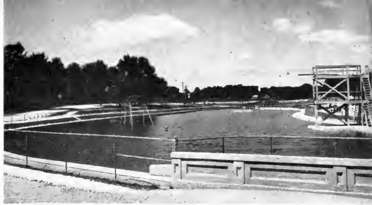
What NOT to do! Features of this pool to be avoided include irregular slope, narrow decks, lights strung up over the pool, too close proximity to a dusty road, and apparatus in pool.
