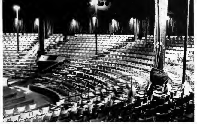
Concrete amphitheatre seats rise in tiers from, and three-quarters around, projecting stage apron. At left is ramp.
