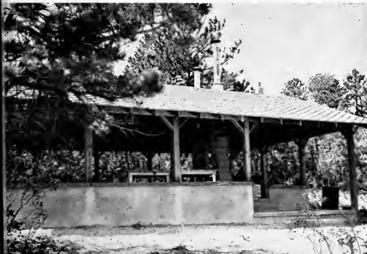
The kitchen and dining pavilion, seen from the hillside, is centrally located. Low wall serves as seat. Eaves extend to form a protection for the open sides.
