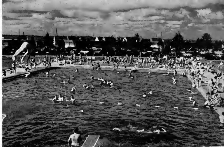
Scene at a Levittown swimming and wading pool clearly illustrates popular use of deck space and of the shallow water area.
