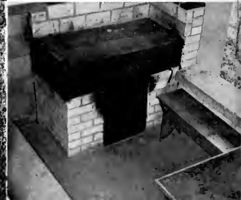
The cooking unit in Rotary shelter is similar to those in dining pavilion. All are enclosed, wood-burning, have ovens.
