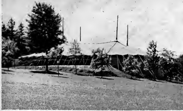
Inner, outer tents make theatre canopy. Weatherproof multiple walls and ceiling assist ventilation and acoustics.
