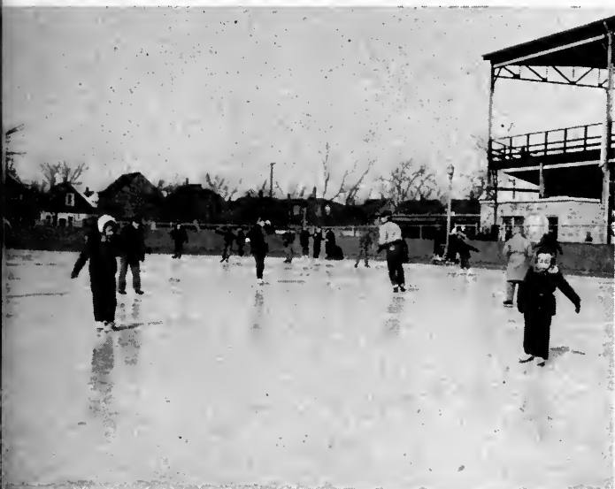
Metal pipe installation is used in this open-type rink in Hamtramck, Michigan. It can later be converted into a concrete all-purpose area for varied year-round activity.
