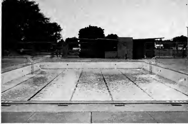
Ready for Business. Brand new Puritas Pool is filled for the first time. Each of these "neighborhood" pools cost $100,000, measures 75 by 42 feet, has a depth range of three to five feet. In the background are facilities for taking showers plus a first-aid room. Note the space at sides of the pool, ample room for sunbaskers.
