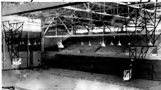
These two Porter 2178 Forward-Fold "Hoistaway" installations were the answer. When not in use the backstops may be hoisted to a horizontal position, permitting overhead room for other activities in the gymnasium.
