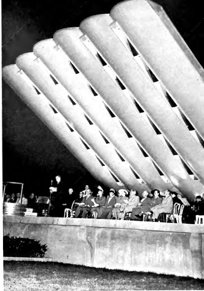
Detroit bandshell sounding board involves a new principle of acoustics, projects sound in equal volume to all audience sections.
