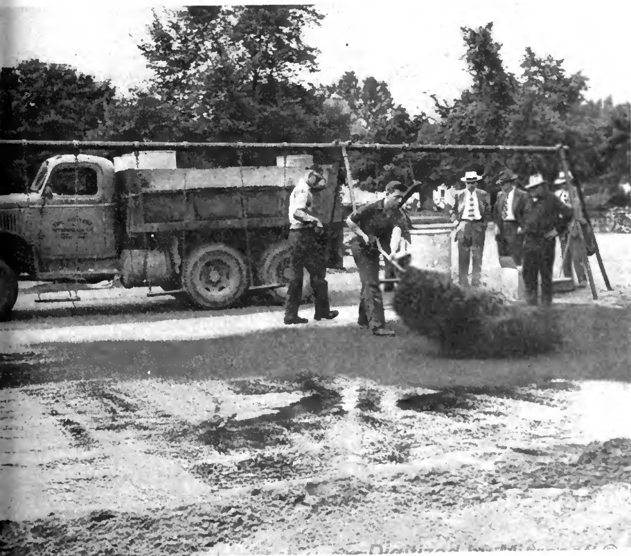
Pelletized rubber is manually distributed over the asphalt binder. Note granular nature of the rubber.
