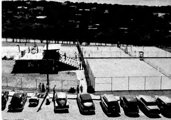
Courts three parts limestone, one part red clay, provide fast-drying excellent play surfaces. Grandstand seats two hundred spectators.
