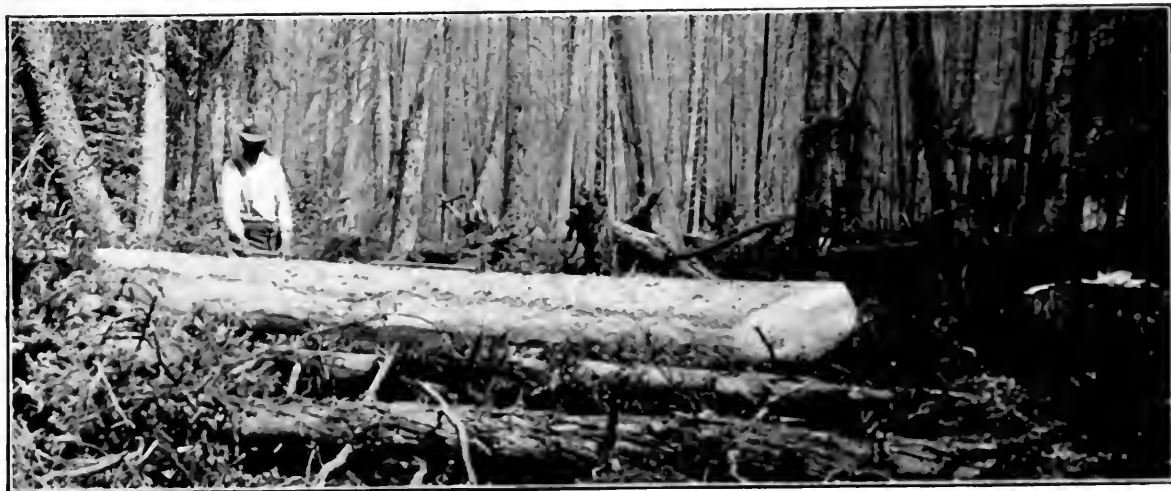
STARTING IN TO EXCAVATE THE HULL.
